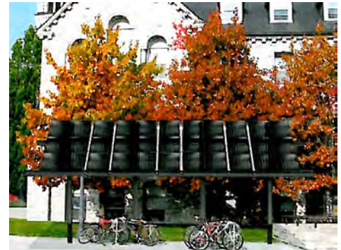
This project of a bicycle shelter at Queen's University with photovoltaic panels on the roof is a simple way to introduce sustainable features to the campus. The shelter can feed electricity back to the grid for 30 years.
