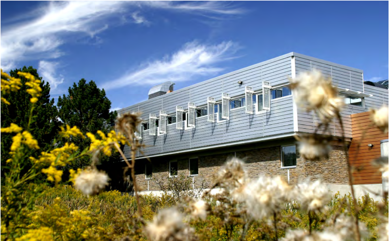
South side of Main Building towards Brealey Woods
