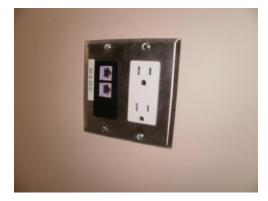
Low density installations in and around legacy installs must be situated either 1000mm/39" of an electrical outlet installed at the same level as associated outlet and have a matching cover plate, or co-located
