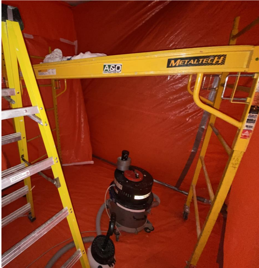
Photograph 2: View of the worker area and enclosure following Type 2 Operation procedures.
