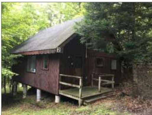
Photo 1 - Cabin 2, 1225 Grass Lake Road.
