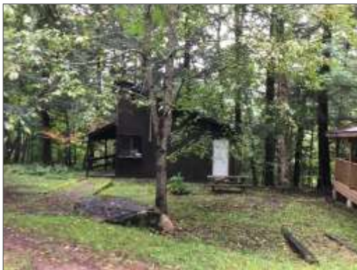
Photo 19 - Cabin 8 at 1225 Grass Lake Road.
