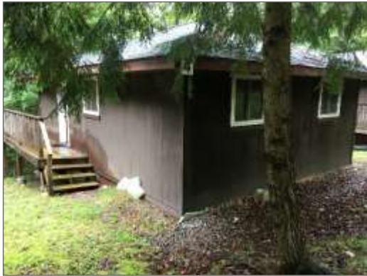
Photo 7 - Cabin 4, 1225 Grass Lake Road.
