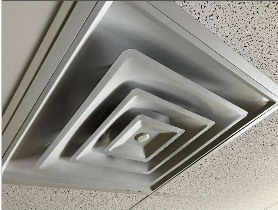
Photo 1 - Diffuser in Office C2147
