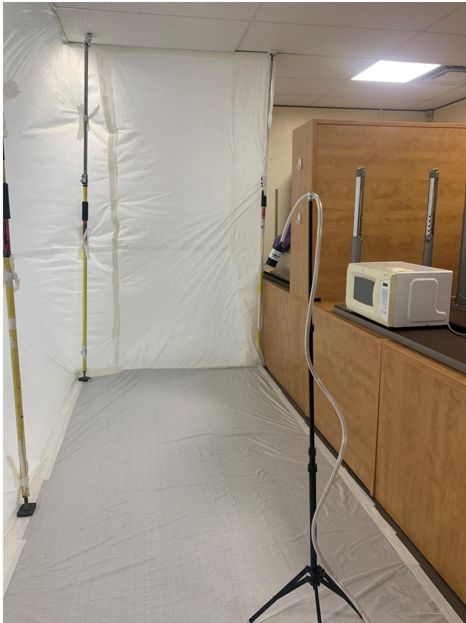
Photograph 2: View of the air sample outside the enclosure of room B2 120.
